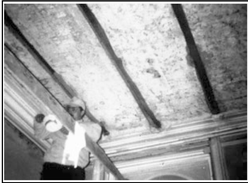
Figure (4.5) – Application of CarboDur laminates
