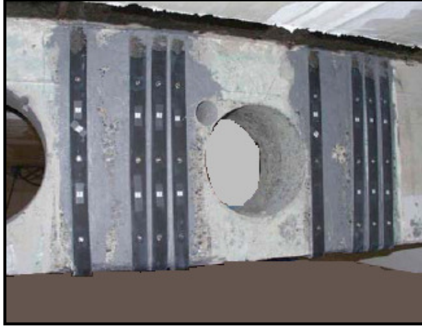
Figure (4.6) – Application of CFRP plates
