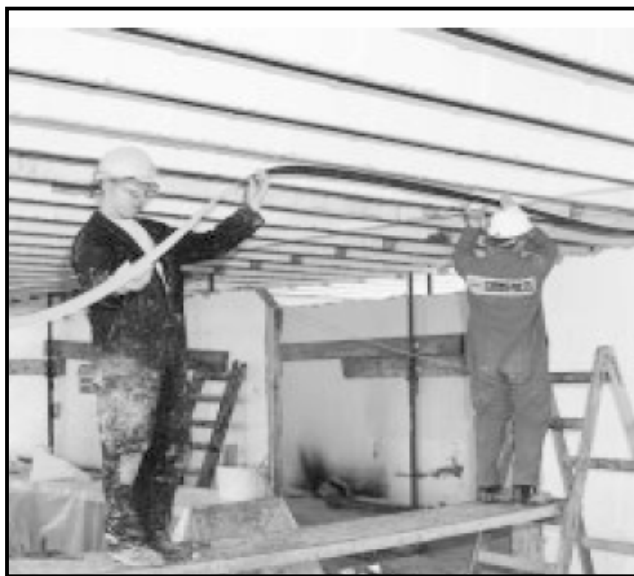
Figure (4.2) – Positioning an 11.0 m laminate to underside of rib (Shaw, 1997)
